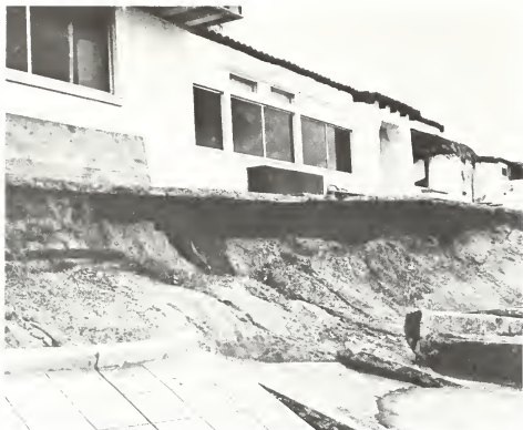
FIGURE 150.—Detail of destruction of the concrete walkway and driveway at Capistrano Beach Club resulting from erosion and attrition of the underlying foundation materials by storm-amplified perigean spring tides occurring around the 1962 February 5 date.
